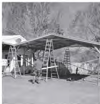
A carport was constructed at the host residence
