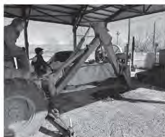
Blair Shean & Bill Allen begin excavation for the Fairbanks Morse engine base
